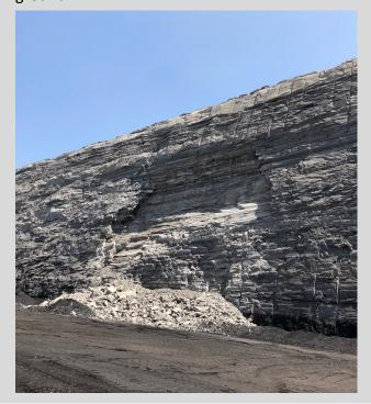
Mine operators must have safe systems of work in place to inspect highwalls. These inspections must consider weathering effects, ground water and conditions that affect the high wall stability.
