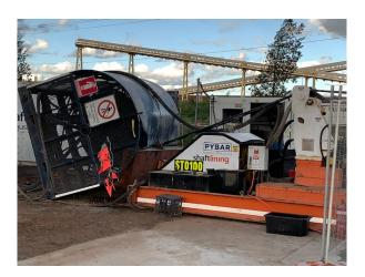
Plant that has the potential to move under strain should be secured in position where possible.
