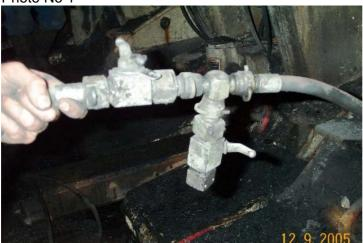
Normal isolation valve and bleed valve arrangement for the Whip Hoses
