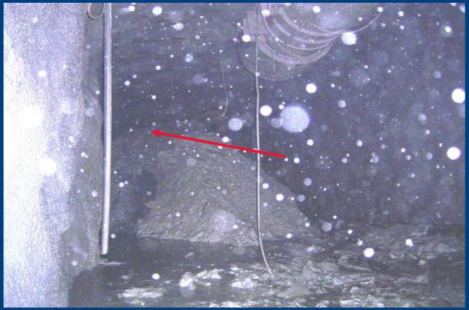
The inrush washed away part of the mound of material and the brattice and consequently changed the ventilation in the mine.
