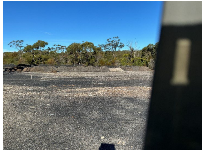
Figure 2 Soil stockpiles opposite North Cliff shaft
