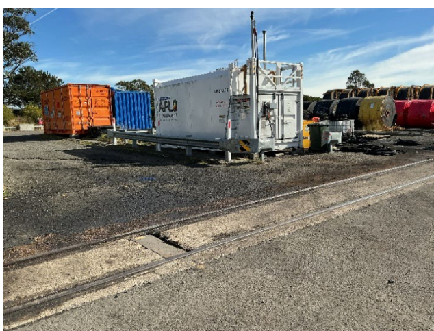
Figure 10 Self-bunded diesel storage
