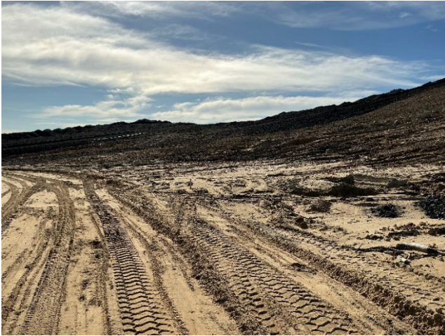
Figure 13 Emplacement area for capping
