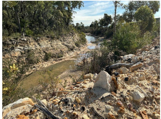
Figure 14 Clean water diversion channel discharging to Brennans Creek
