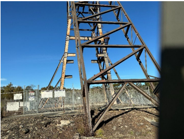
Figure 1 North Cliff shaft number 4
