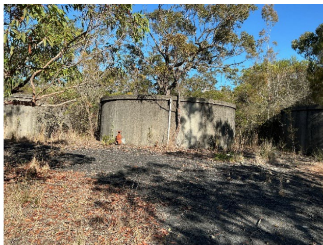
Figure 6 Decommissioned concrete tanks at North Cliff site
