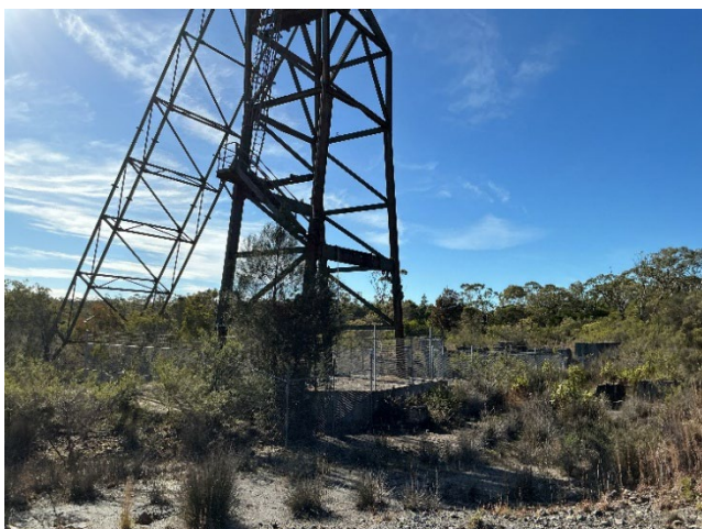
Figure 5 North Cliff shaft number 3
