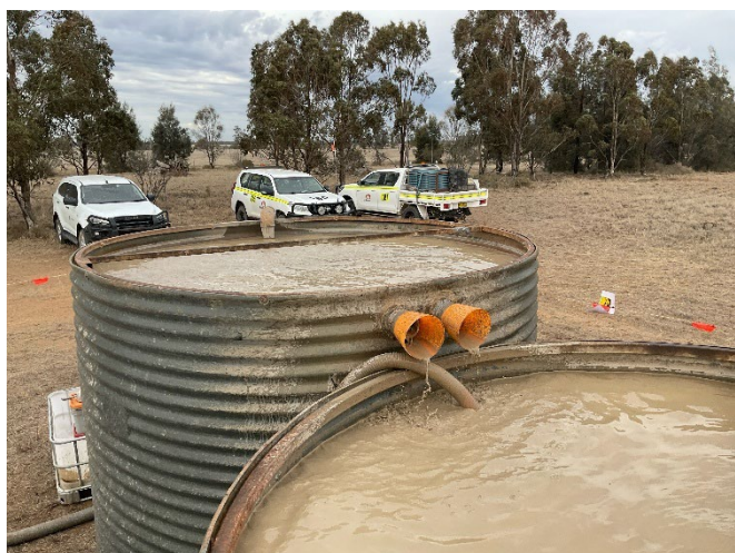
Figure 9: Erosion and sediment controls on a drill pad
