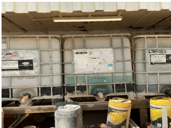
Figure 25: Bunded and covered chemical storage
