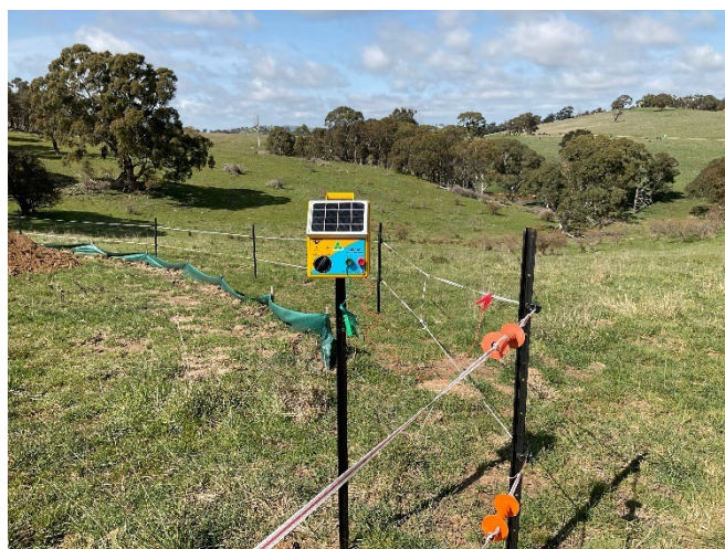
Figure 10: Electric fencing around drill pad
