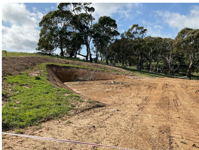
Figure 9: Erosion and sediment controls on a drill pad
