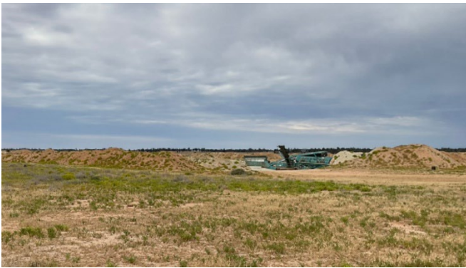
Figure 4: The processing plant in the current mining operation area
