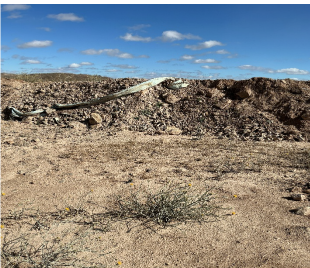
Figure 5: Not properly installed sediment fencing
