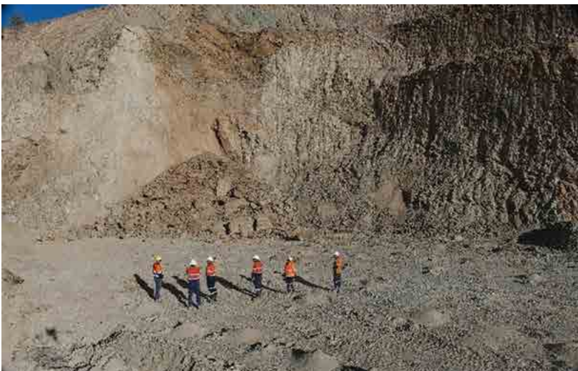
Picture 1. Wall failure above sleeping shot.
