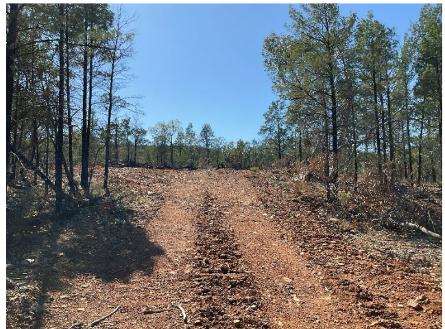
Figure 2: Surface disturbance and vegetation clearance associated with access track to drill pad YMRC003
