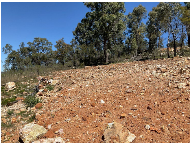
Figure 6: Reshaping and initial rehabilitation of low grade east bulk sample pit on EL5920
