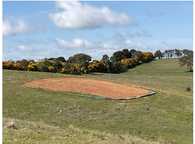
Figure 18: Initial rehabilitation of diamond drill hole X059 drilled in August 2025
