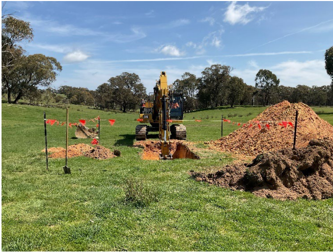
Figure 12: Typical surface disturbance associated with costeaning operations
