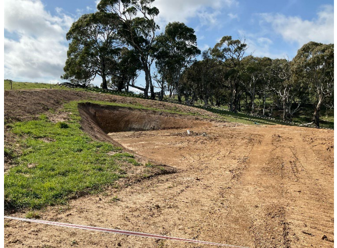
Figure 11: Sediment fencing downslope of reshaped drill pad for hole X043 drilled in August 2025
