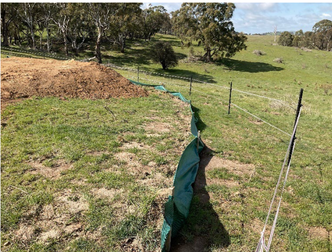
Figure 10: Sediment fencing downslope of hole X060 drilled in September 2025
