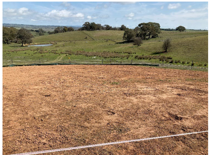
Figure 11: Sediment fencing downslope of reshaped drill pad for hole X043 drilled in August 2025
