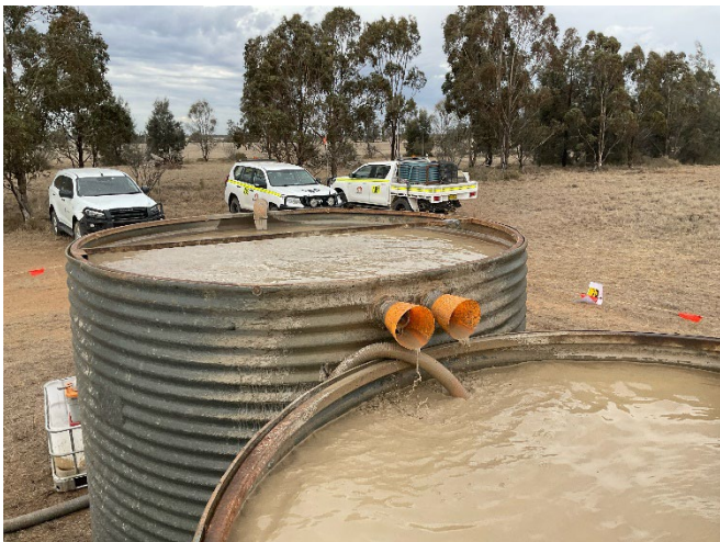
Figure 3: Aboveground sumps used for drilling water management
