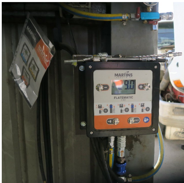
Figure 6: Inline pressure gauge fitted to compressed air line system
