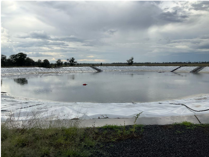
Figure 3: Lined produced water management pond at Tintsfeld
