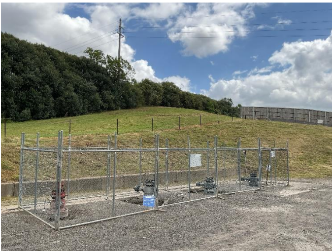
Figure 3: Wells Menangle Park 1, 2, 3 and 9 - all wells plugged and decommissioned awaiting cut and cap
