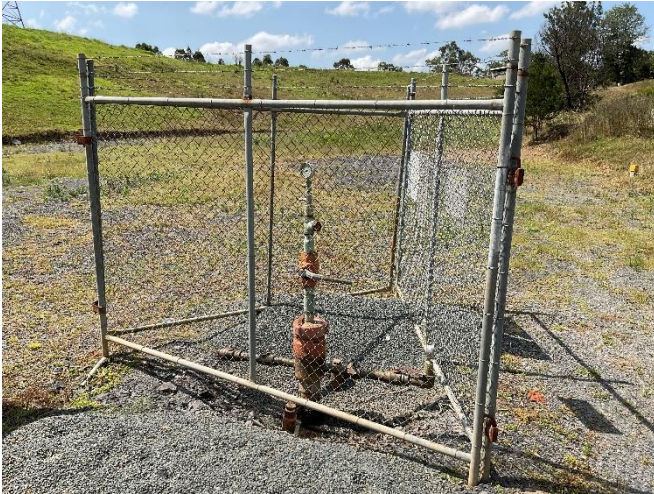
Figure 3: Wells Menangle Park 1, 2, 3 and 9 - all wells plugged and decommissioned awaiting cut and cap
