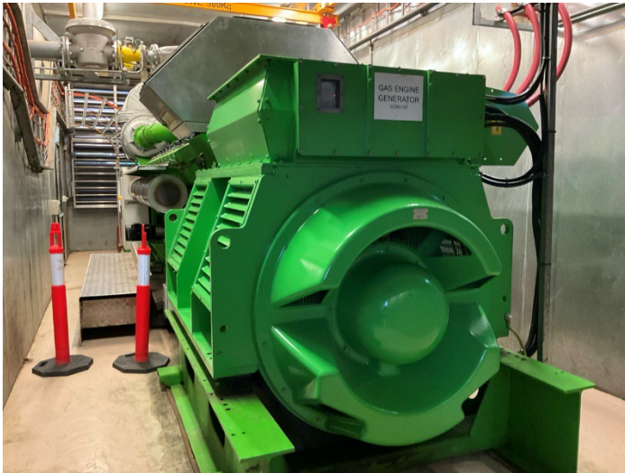
Figure 14: A gas fired engine generator at the Wilga Park Power Station
