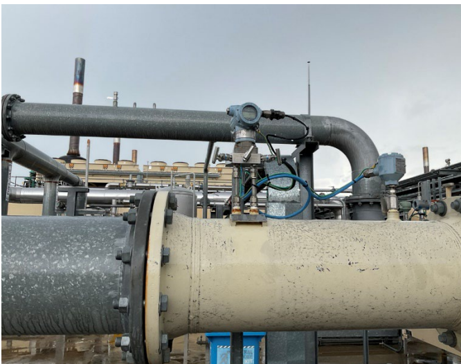
Figure 15: Metering of gas inflows to the Wilga Park Power Station
