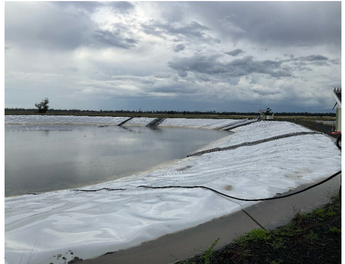
Figure 3: Lined Pond 1 at Tintsville produced water management facility
