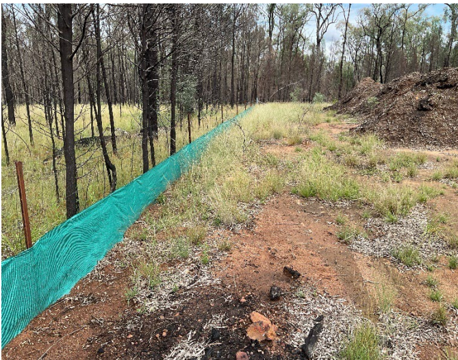
Figure 6: Sediment fencing and mulch piles for partial rehabilitation at Dewhurst 28
