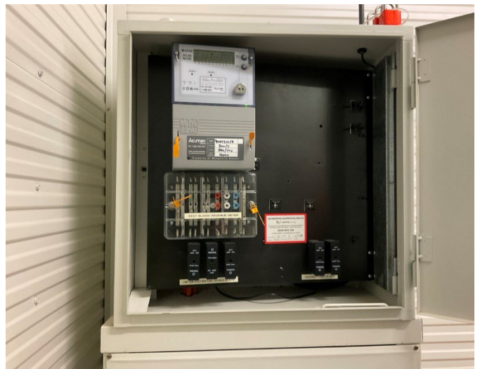
Figure 16: Metering of energy produced from the Wilga Park Power Station
