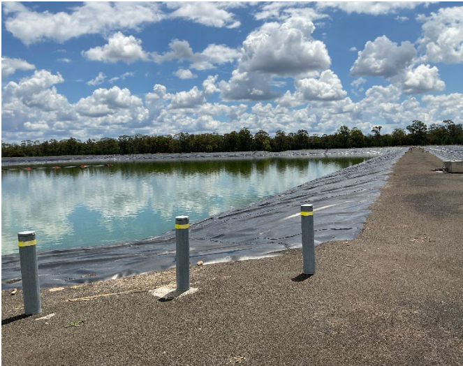
Figure 2: Lined pond at Leewood produced water management facility
