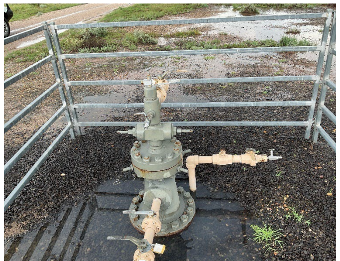
Figure 13: Handles locked or removed at Wilga Park 1
