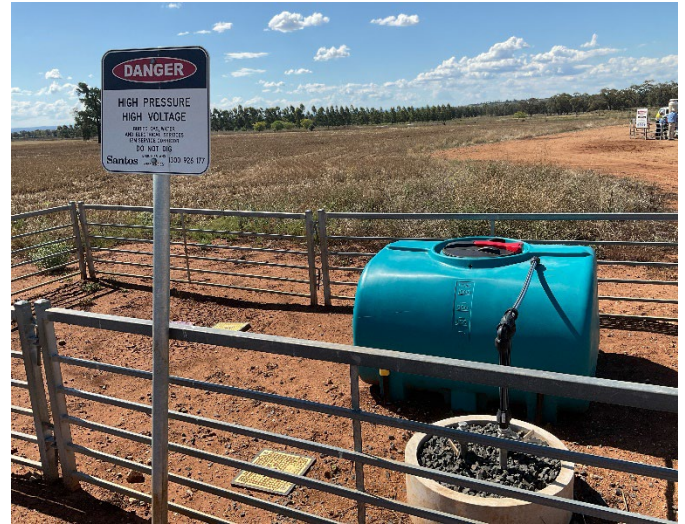
Figure 4: Stock fencing around a low point drain
