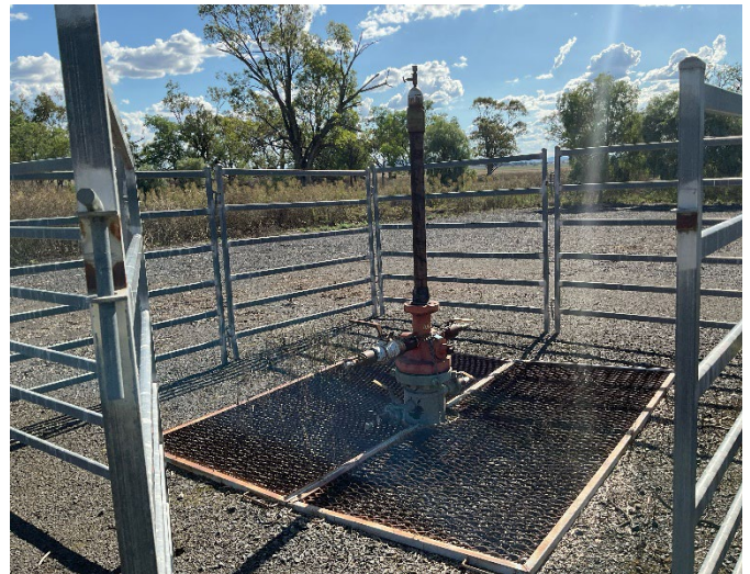
Figure 9: Wellhead valves chained and locked at Longlea 1
