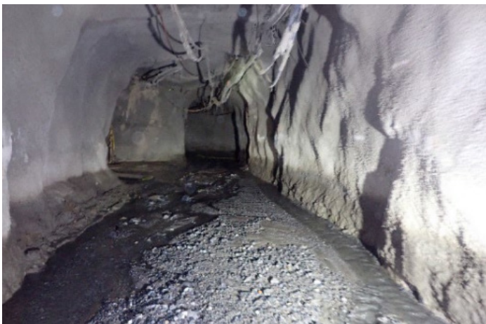
Picture 4. Damp walls indicating the water level reached
