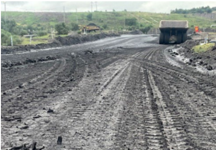
Picture 11. Truck stopped at windrow after traction loss
