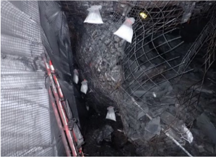
Picture 3. Roof failure impeding access
