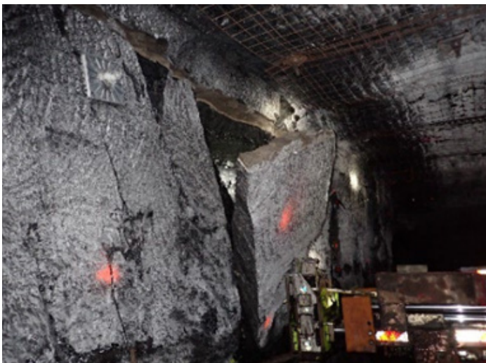
Picture 1. Rib slump in panel
