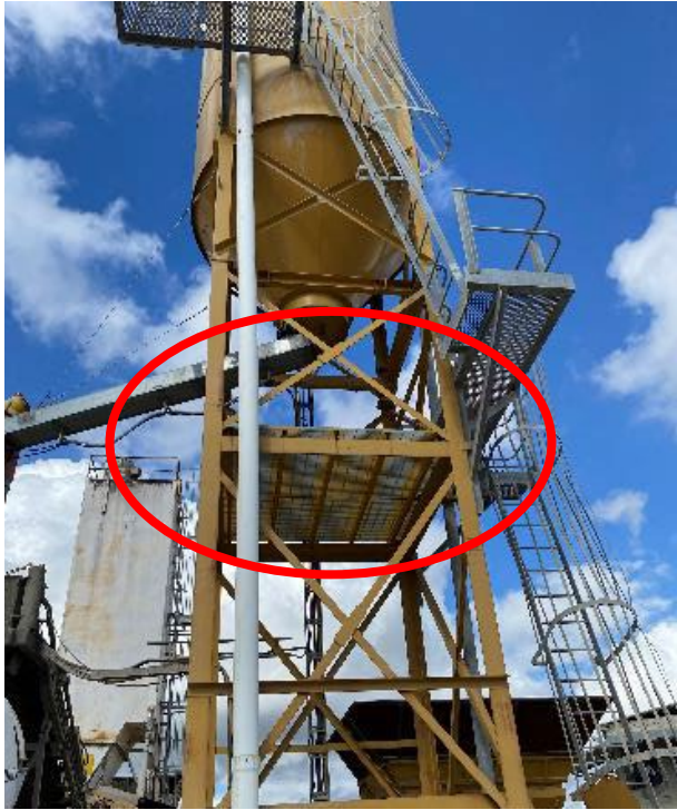
No fall protection on platform
