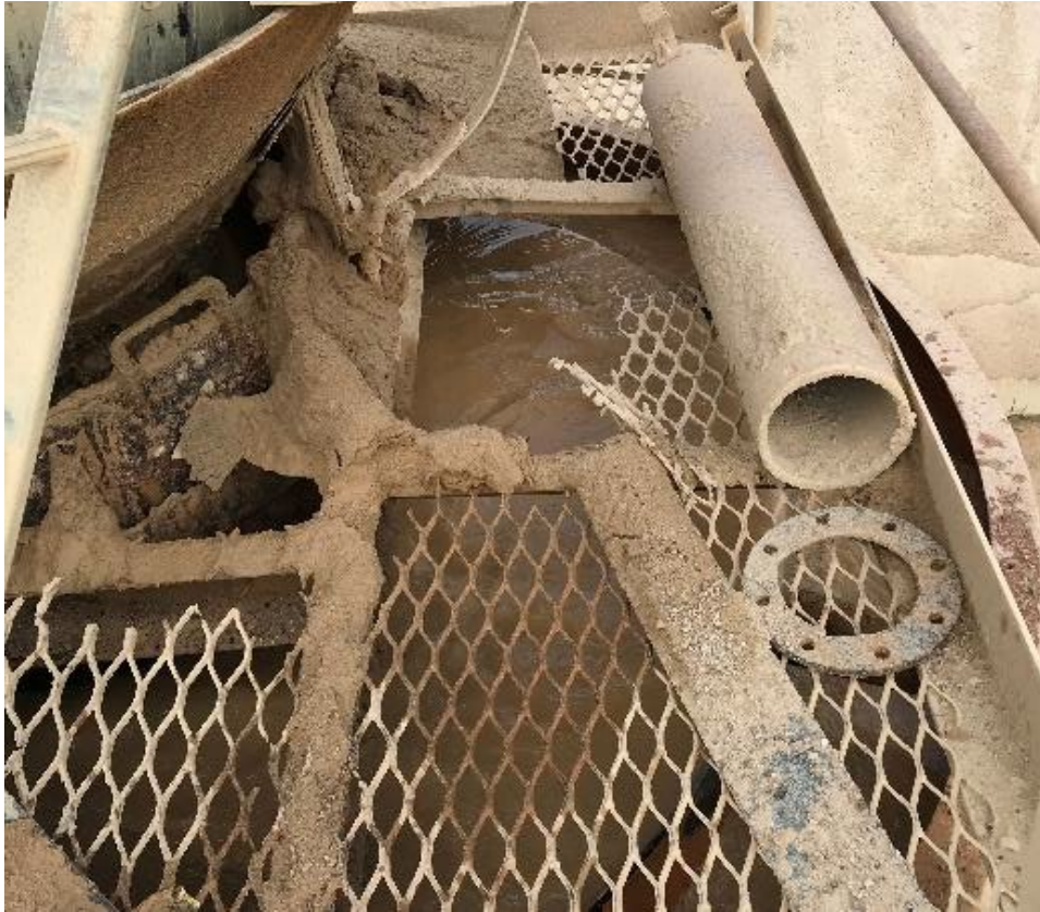
Heavily corroded grid mesh
