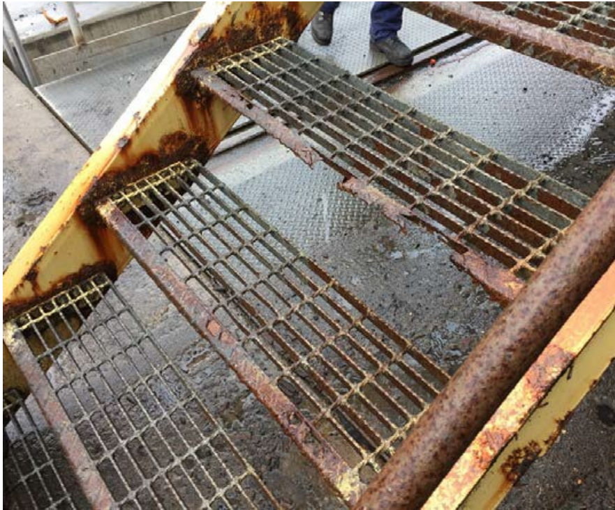
Heavily corroded walkway treads
