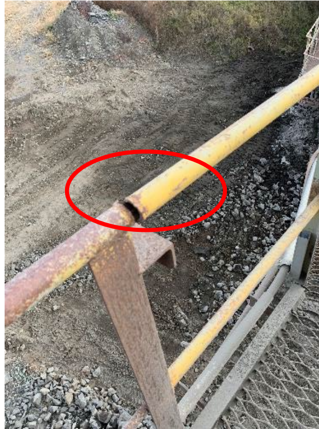
Cracked handrail
