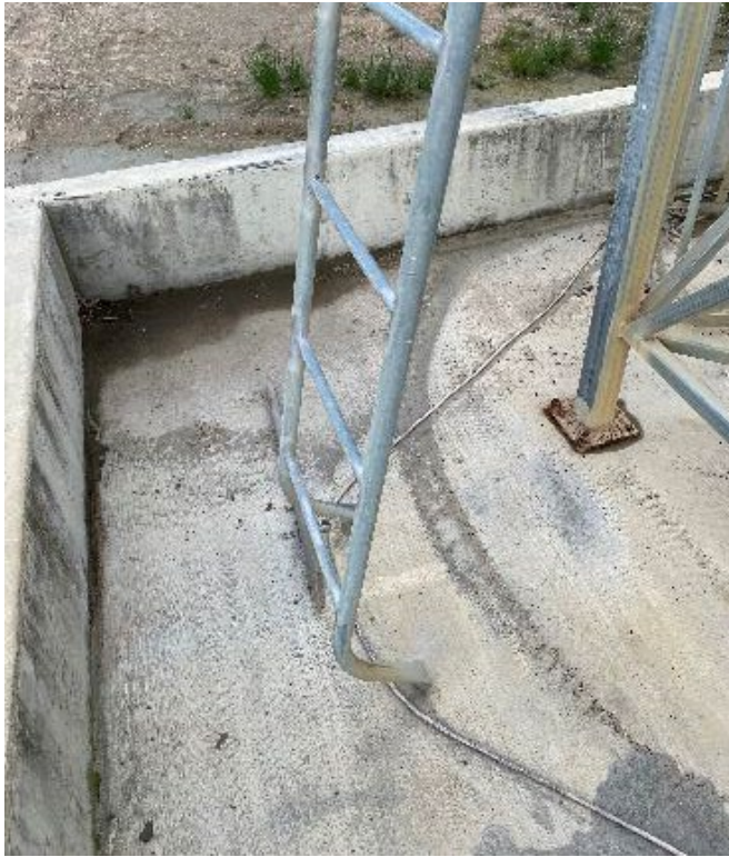
Ladder base not secured
