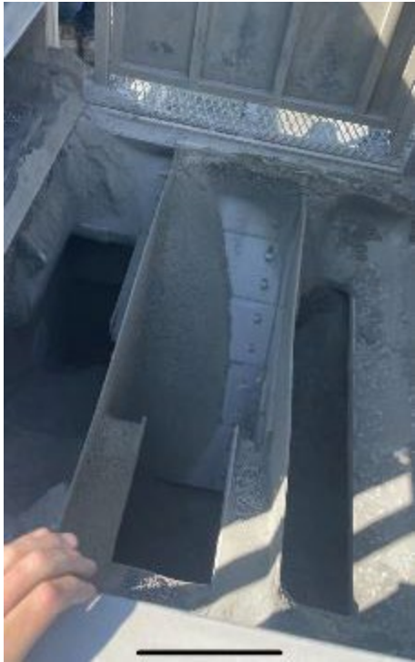
Chute cover moved but platforms still prevent worker access to fall zone
