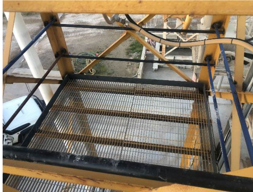
Handrails and kickplates fitted around the platform. Kickplates also help to provide containment for dropped tools.
