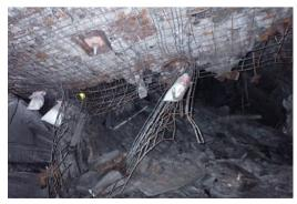
This incident highlights that loading applied to an active tailgate roadway ground support increases immediately outbye the faceline as the face retreats and abutment loads are redistributed outbye. This increase in loading on the installed ground support, particularly if accompanied by the presence of a localised geological anomaly can result in a fall of ground.
