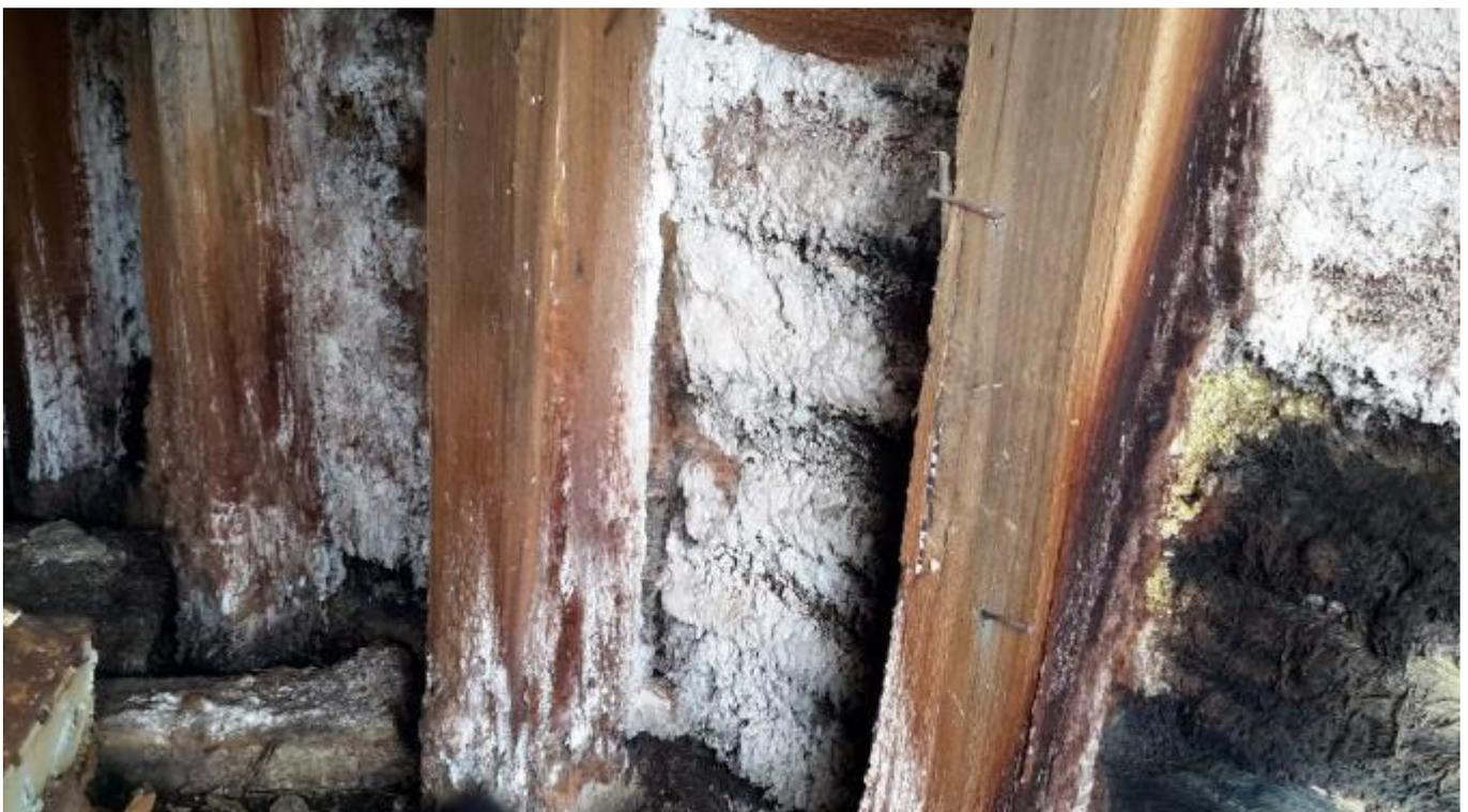
**Figure 4.4**      *Sulfate efflorescence in central Concentrate Loading Tunnel*
