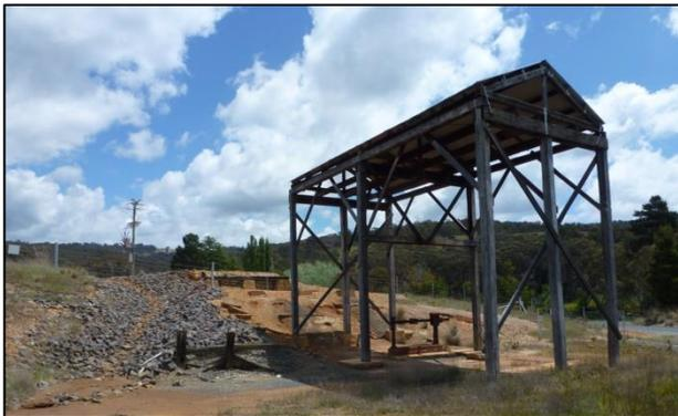
*Figure 4.1 Weighbridge (reconstructed from original and new materials following unauthorised demolition). Image: GHD 2022*
