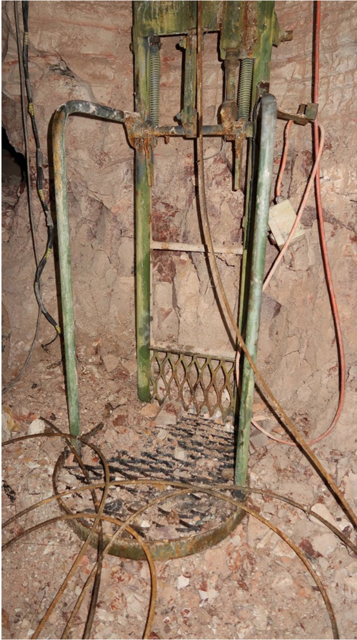
Figure 3: Person riding hoist found at the bottom of the shaft with unspooled cable. Note the safety breaking system has not engaged
