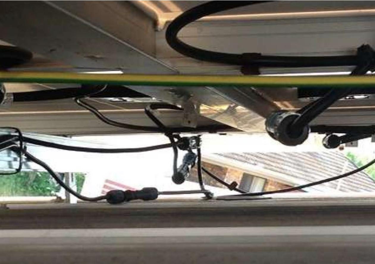
DC Cable installation non-compliant to AS/NZS 5033 resting & rubbing on roof
