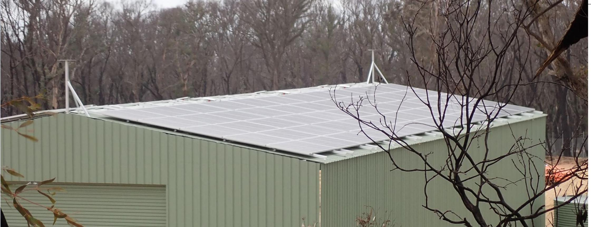
Off grid system – 120 cells (3 phase system with batteries and a generator back up)
