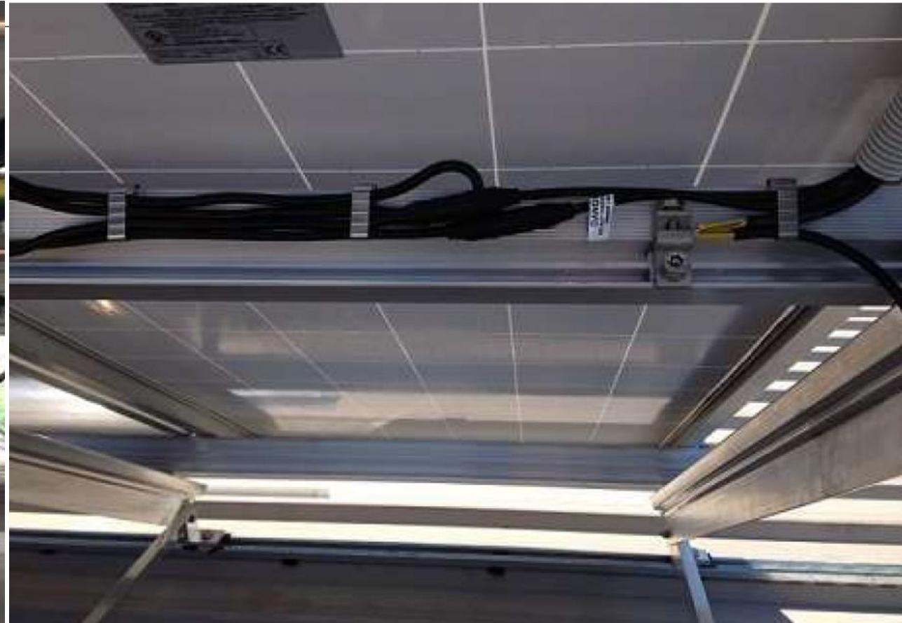
DC Cable installation to compliant to AS/NZS 5033 stainless clips & out of sunlight
