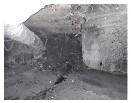
3. In a development roadway, a strata failure occurred 60 metres behind a continuous miner moments after a shuttle car passed through the area where the fall occurred.
